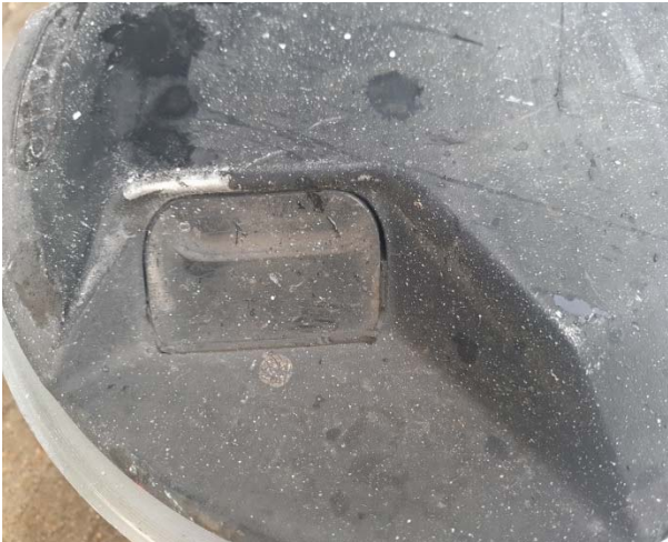
Fig. 1 Before dry powder blasting
