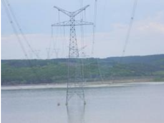
Figure 4 Installation environment of aeolian vibration on-line monitoring system in Hemu Line B.
