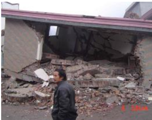
Fig 9 Integral collapse of brick-concrete structure of bottom frame
