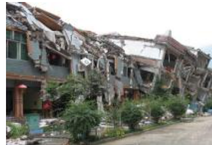
Fig 13 The collapse of a three-story frame structure in Beichuan County
