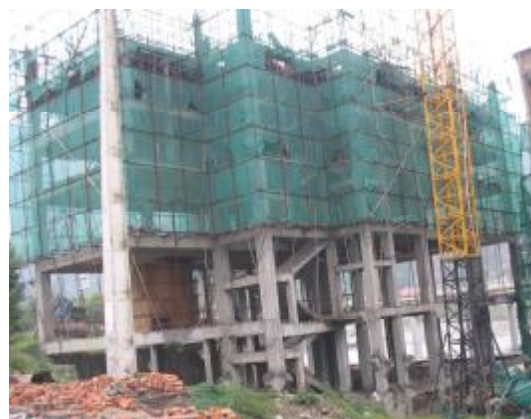
Fig 9 Integral collapse of brick-concrete structure of bottom frame
