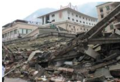
Fig 12 Partial collapse of Beichuan Hotel
