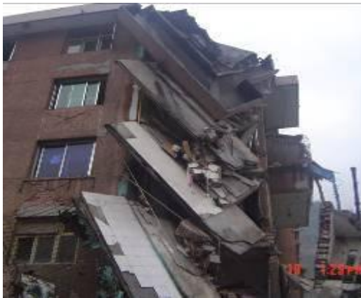
Fig 7 Domino effect triggered by prefabricated slabs
