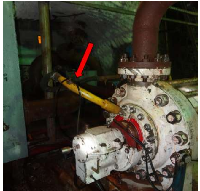
Fig. 10. Unloading pipe of the JSH-200 section pump produced by Mackley Pumps
