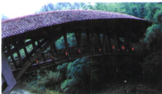
Fig. 7. Shizishui bamboo bridge.
