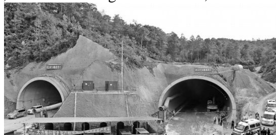
Fig.1 Highway tunnel in mountain area of Guangshan No.1 tunnel
