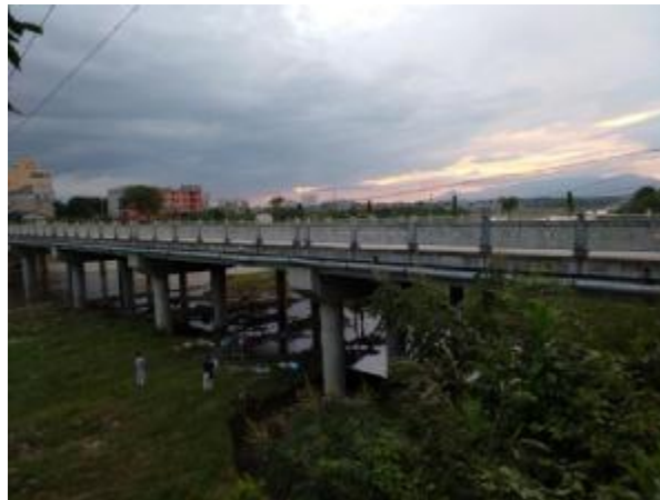
Fig. 1 The full view of Chang pugang Bridge
