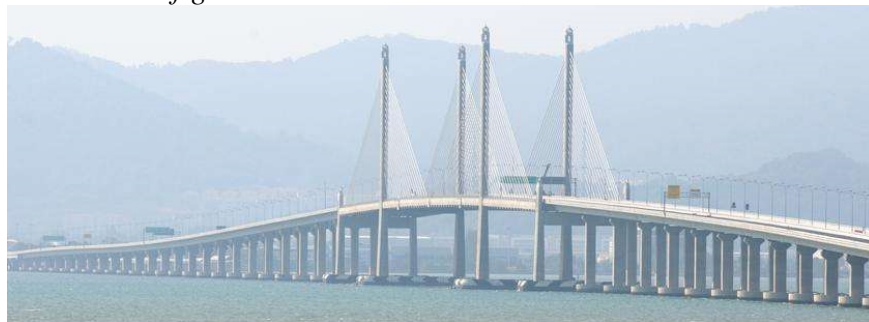
Fig.1 General view of Penang Second Marine Bridge.
