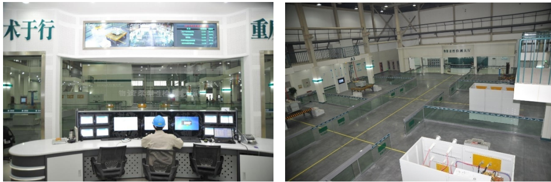
Fig. 1. Large screen display system and flexible detection hall in State Grid Jiangsu Electric Power Research Institute
