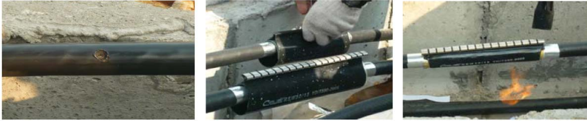
Fig.3 Method of using cable patch.
