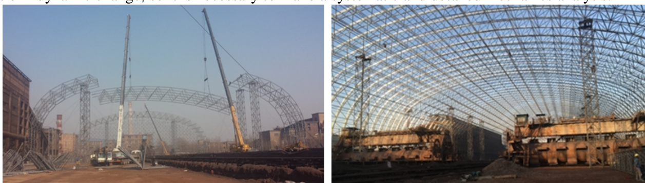
Fig.2 The layout of the temporary support frames
