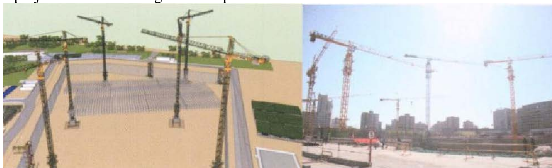
Fig. 3 Comparison of BIM Construction Site Arrangement Model and Actual Construction Site Photographs
