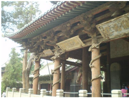
Fig. 2. Shanxi province taiyuan Jinci goddess hall façade.
