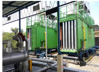
Figure 1. One of waste processing machine on LPA Benowo, Surabaya
