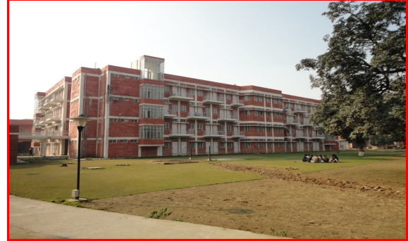
Fig.1 Data collection site building
