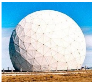
Fig.1 Metal space frame radome
